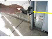
NOT AUTO REVERSING BY PRESSURE: The garage door automatic opener is not automatically reversing when physically blocked by the inspector – correction/adjustment is recommended. Contact a contractor for evaluation
